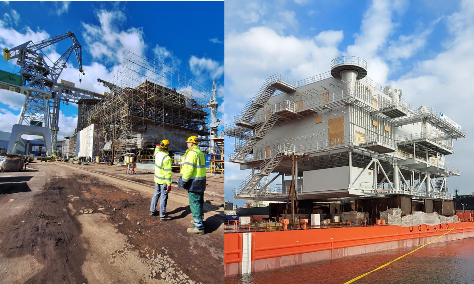
Prefabrication of two substations (OSS), 2 x 1150 tons for American OWF
